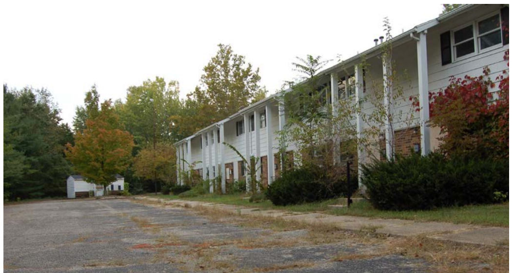
Abandoned site ripe for redevelopment
