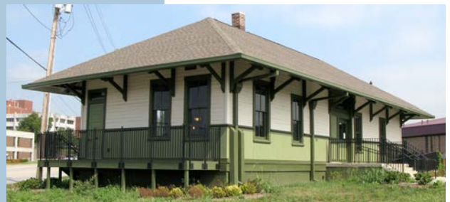
The National Register-listed Spring Street Freight House (c.1925) in Jeffersonville, Indiana, was recently rehabilitated for office use and remains a neighborhood landmark
