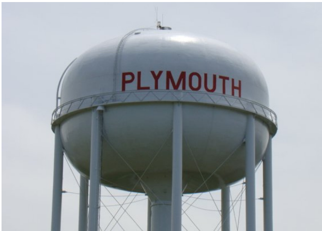
One of Plymouth's water towers, located in an industrial park.
