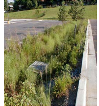
Stormwater best management practices include rain gardens and permeable pavement. Application of such techniques minimizes stormwater runoff.
