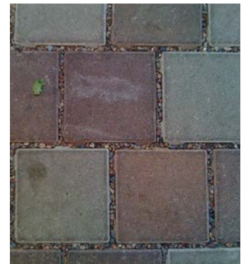
Stormwater best management practices include rain gardens and permeable pavement. Application of such techniques minimizes stormwater runoff.
